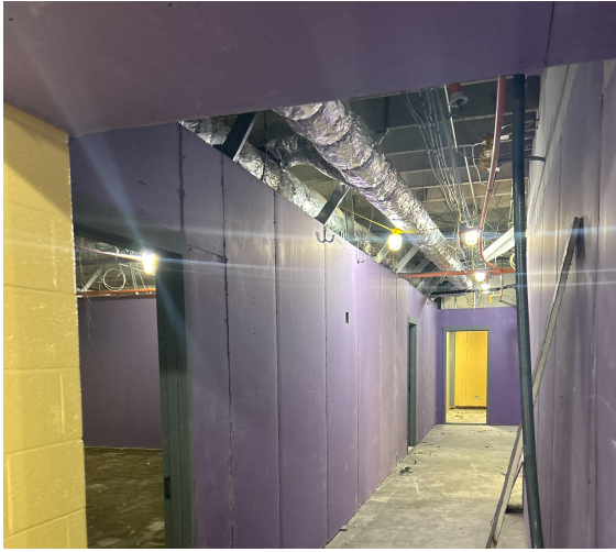
Dry wall installation in the classrooms on level 2.
